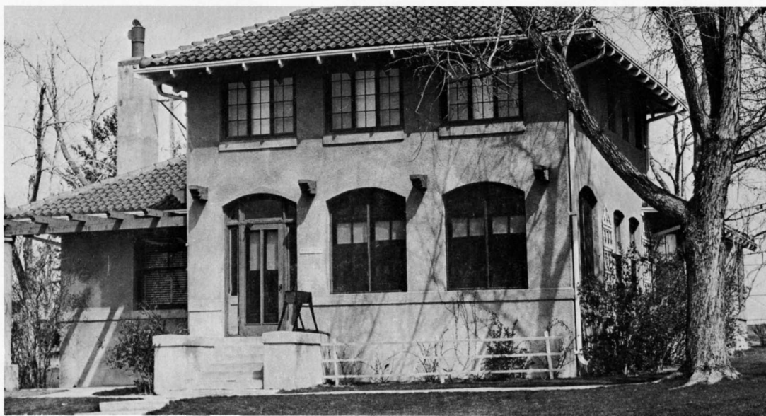
Building 251, dating from the Agnes Memorial Sanitorium, has been the home of many Lowry commanders.
