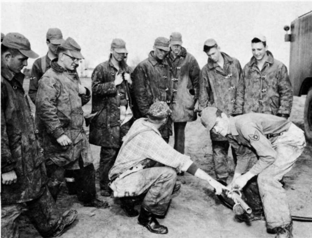
Students from the Department of Fire Protection and Aircraft Rescue Training practice using a hand spray nozzle and foam sprayer equipment.
