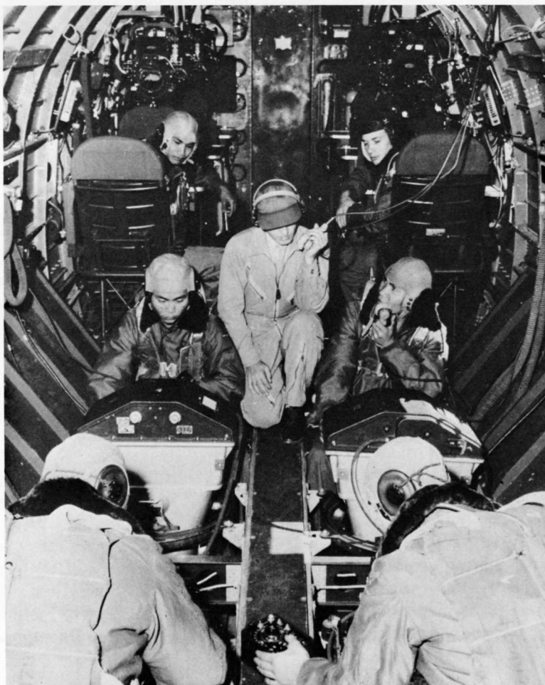
In October 1943 the Army transferred the Flight Engineers School to Lowry. This 1945 photograph shows a B-29 flight engineer station and trainer.
