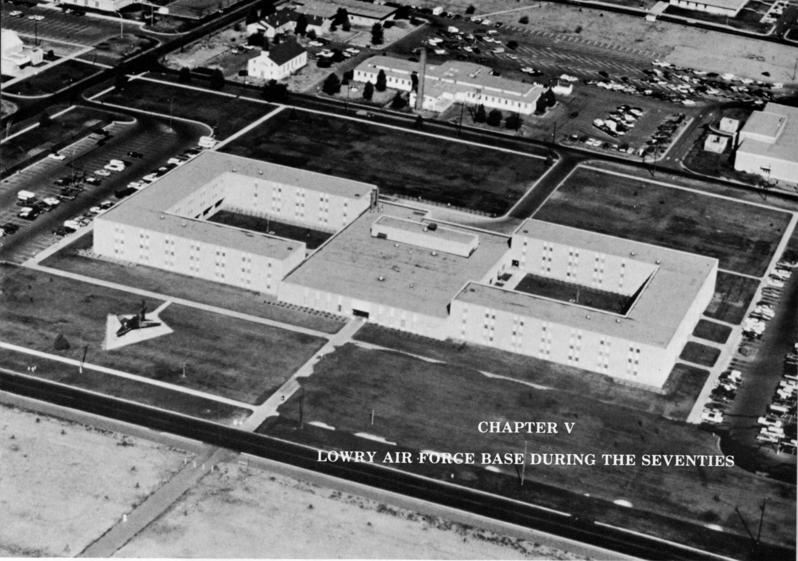
Building No. 700 was one of five 1,000-person dormitories constructed during the 1970s.
