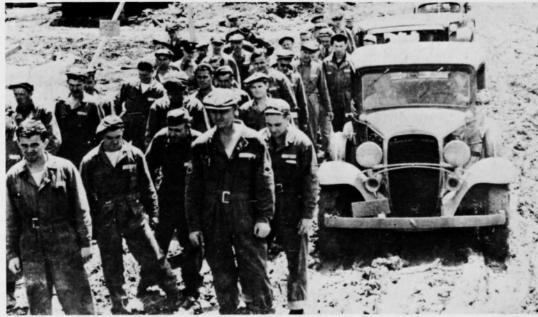
During the early years at Lowry, funds had only been appropriated to renovate existing structures and erect new buildings. Road construction did not begin until December 1940.
