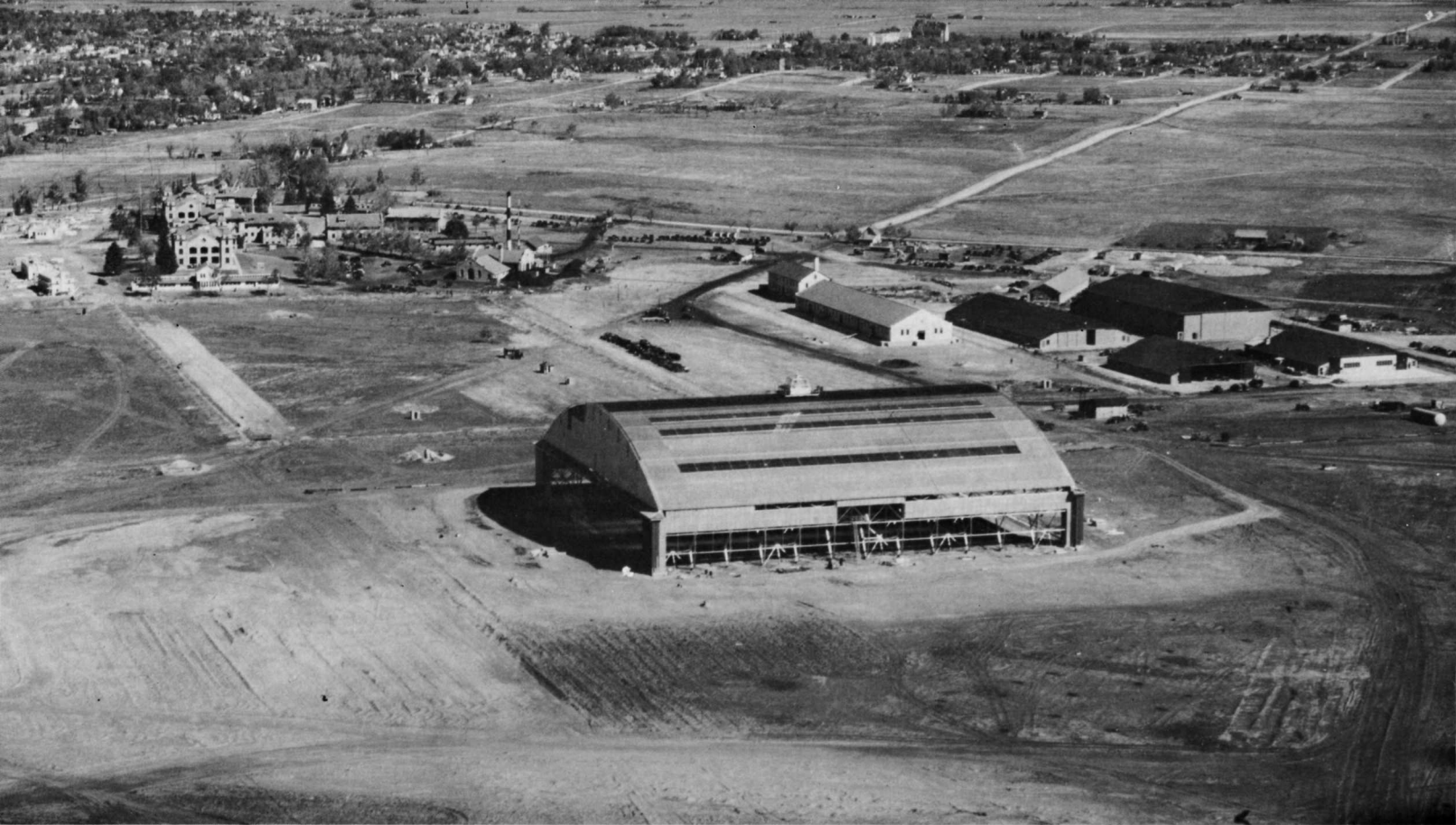
Construction of Lowry's first large hangar began in 1939. In December, the Air Corps moved its flying and maintenance activities inside even though the facility still lacked lights, heat, and hot water. The intensity of the cold and the need to wear winter clothing aggravated working conditions. In January 1940 the Quartermaster put stoves in the hangar until steam heating units could be installed.
