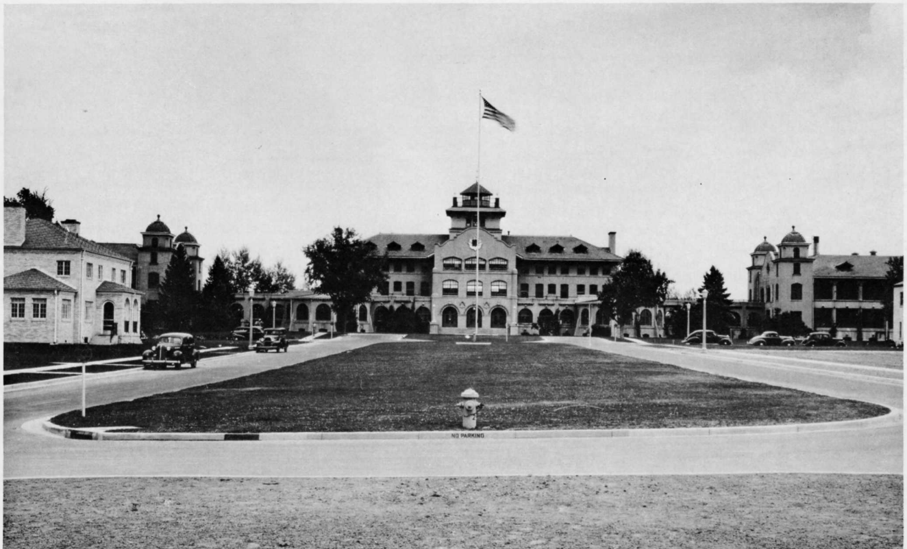
The Army renovated the Agnes Memorial Sanatorium for the Air Corps Technical School. The building in the center of this 1940 photograph was the headquarters for Lowry Field. The new brick structure in the left foreground served as quarters for noncommissioned officers and their families.
